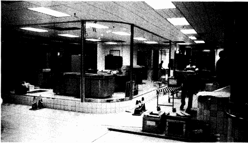
● Moving gear into the Computer Room, a focal point in the customer reception area.
